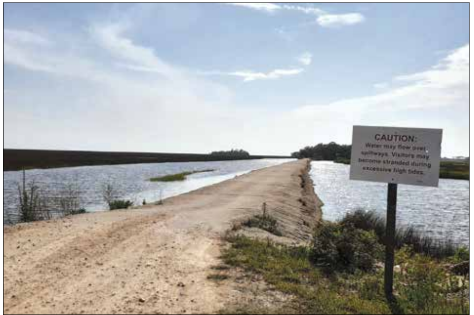
Bridge roadway leading across the marsh tides
